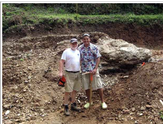
Steve and Alex breaking rock
